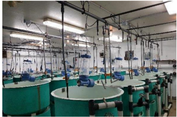
Figure 9. Photo showing the White Lake FCS's Lake Whitefish early rearing room equipped with 500-litre conical tanks and Arvo-Tec feeders.
